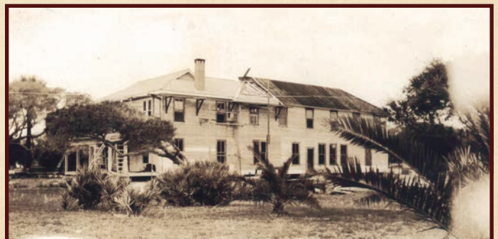
Olivia Gamble's restoration work underway c. 1938. Collection of the Ponce de Leon Inlet Lighthouse Preservation Association
