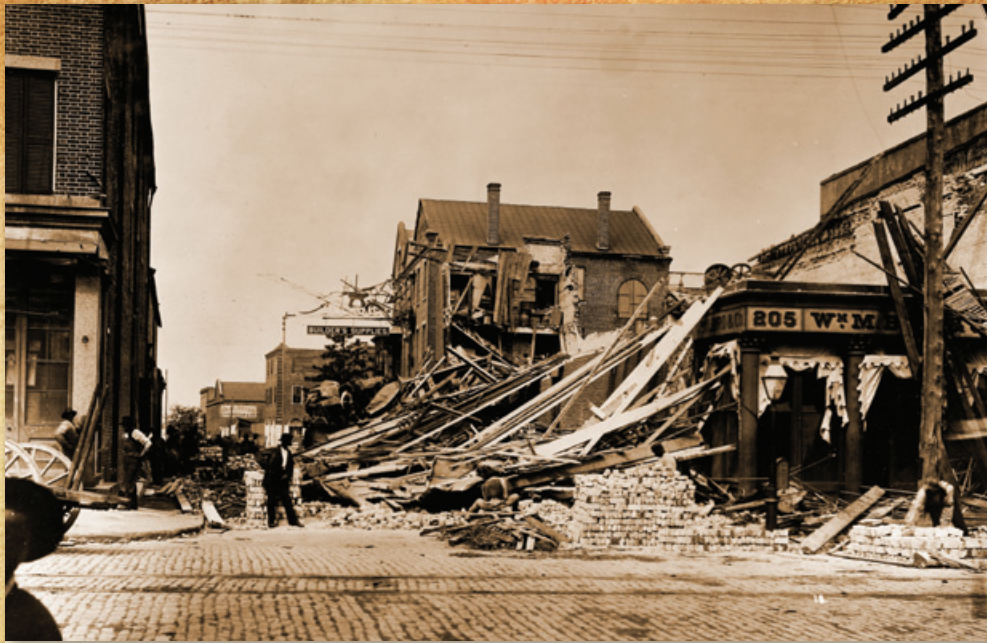
ALL BUILDINGS IN CHARLESTON WERE DAMAGED AND MANY WERE DESTROYED.
