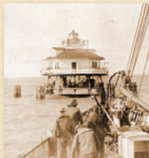
LAUREL POINT LIGHTHOUSE
