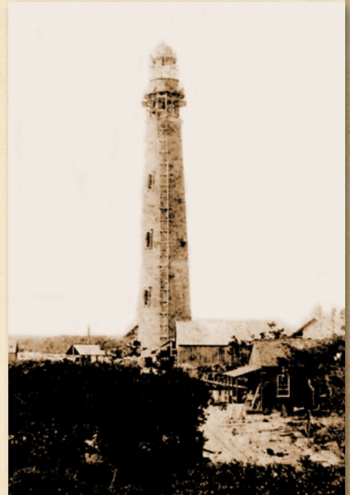
MOSQUITO (PONCE) INLET LIGHT STATION WAS UNDER CONSTRUCTION AT THE TIME OF THE QUAKE
