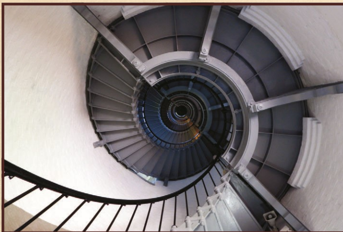
Iron was used in the construction of the lighthouse's spiral staircase as well as its balcony and lantern room. This is a picture looking upwards from the inside of the Ponce Inlet Lighthouse, 2019.
