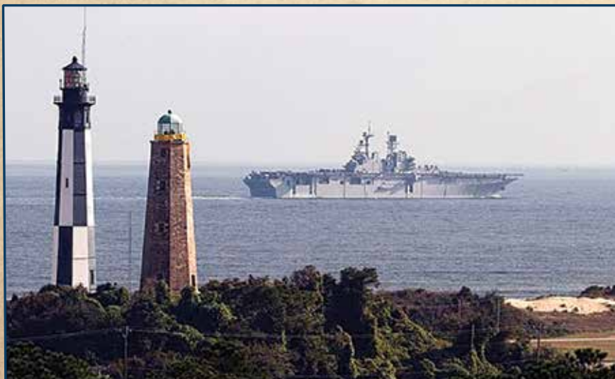
The “Old” Cape Henry Lighthouse constructed during Hamilton's tenure as secretary of the treasury and head of the US Light-House Establishment stands beside its “replacement” the “New” Cape Henry Lighthouse.
