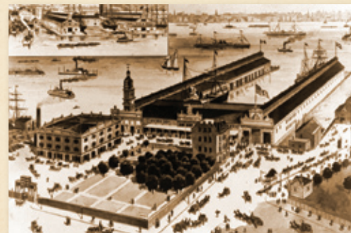
THE ALEXANDRE & SONS COMPANY UTILIZED PIER 3 IN NEW YORK FOR MUCH OF ITS SHIPPING BUSINESS
