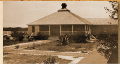
PRINCIPAL KEEPER DWELLING WITH 1921 BATHROOM ADDITION NEARLY COMPLETED
