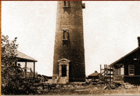
RE-ROOFING THE SECOND ASSISTANT KEEPER DWELLING IN 1907
