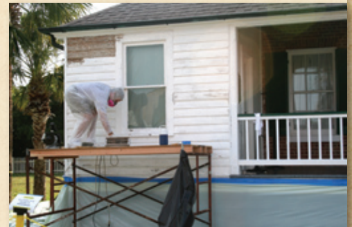
RESTORATION OF PRINCIPAL KEEPER DWELLING BATHROOM ADDITION, JUNE 2010
