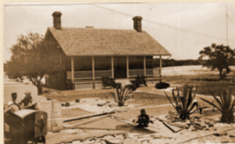
SECOND ASSISTANT KEEPER DWELLING WITH CONCRETE APRON INSTALLATION IN FOREGROUND AND RADIO ANTENNA TOWER IN RIGHT BACKGROUND
