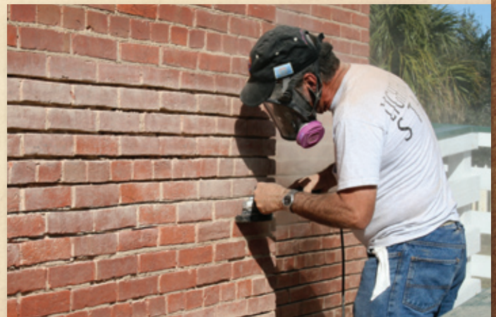
THE FIRST ASSISTANT KEEPER DWELLING UNDER REPAIR IN 2000
