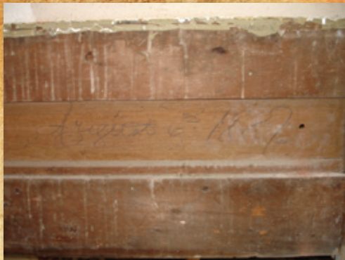
CARPENTER'S SIGNATURE ON LIVING ROOM FIREPLACE MANTEL, SECOND ASSISTANT KEEPER DWELLING
