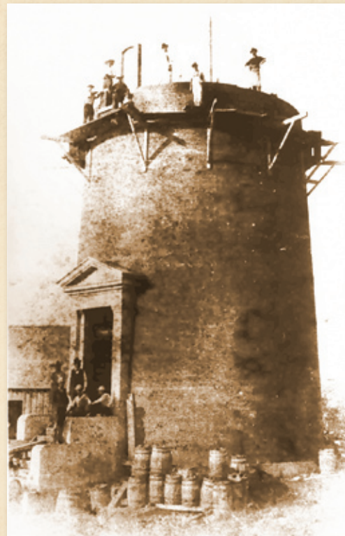
TOWER UNDER CONSTRUCTION
