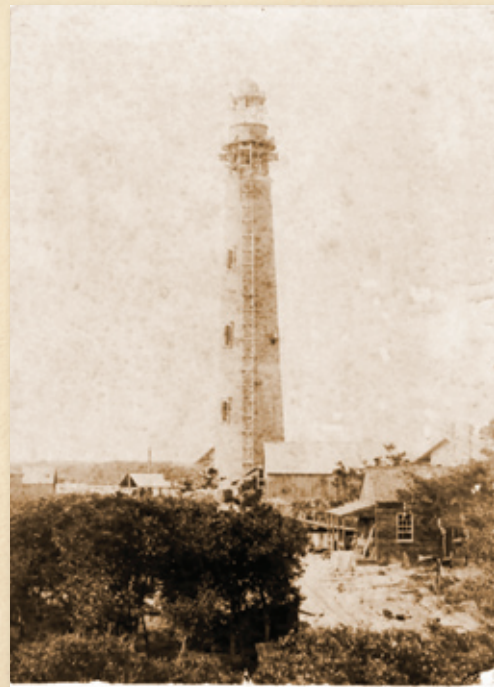
INSTALLATION OF LANTERN ROOM. NOTE HOIST LADDER ATTACHED TO TOWER.
