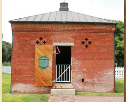
THE RESTORED OIL STORAGE BUILDING
