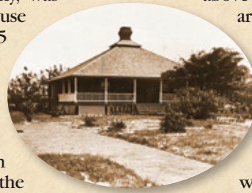
PRINCIPAL KEEPER DWELLING BEFORE BATHROOM ADDITION
