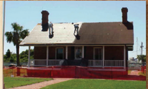
THE FIRST ASSISTANT KEEPER DWELLING UNDER REPAIR IN 2000
