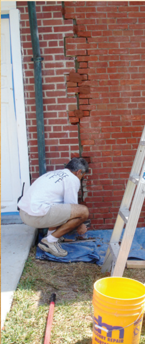
GENERATOR BUILDING MORTAR RESTORATION, 2007
