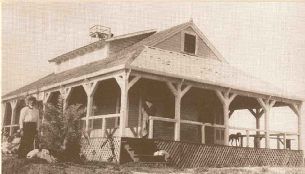
MOSQUITO LAGOON HOUSE OF REFUGE
