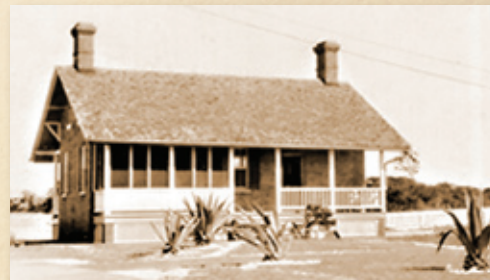
SECOND ASSISTANT KEEPER'S DWELLING AT MOSQUITO INLET LIGHT STATION
