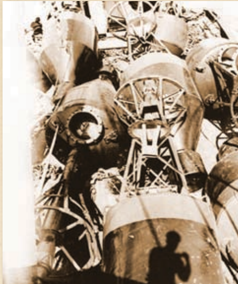
BELL BUOYS, MOORING CHAINS, AND WEIGHTS ("ROCKS") PILED ON THE DECK OF THE USLHT Oak .
