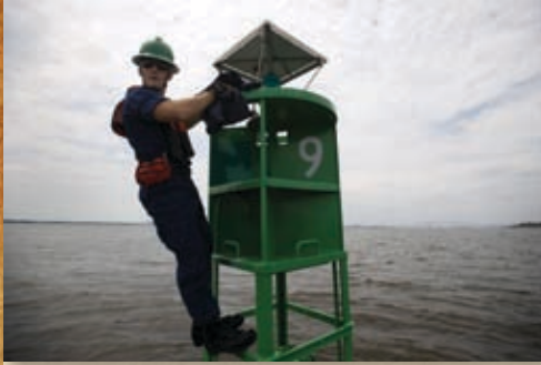
AN ATON COAST GUARDSMAN PERFORMS MAINTENANCE ON THE SOLAR PANEL OF AN ILLUMINATED BUOY.
