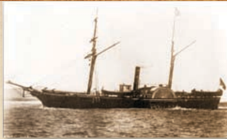
COMMISSIONED IN 1857, THE USLHT Shubrick WAS THE LIGHTHOUSE ESTABLISHMENT'S FIRST STEAM POWERED TENDER. IT SAW SERVICE ON THE WEST COAST.
