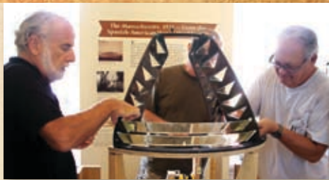
ART HAHN & JIMMIE V. INSTALL AN UPPER CATADIOPTRIC PRISM
