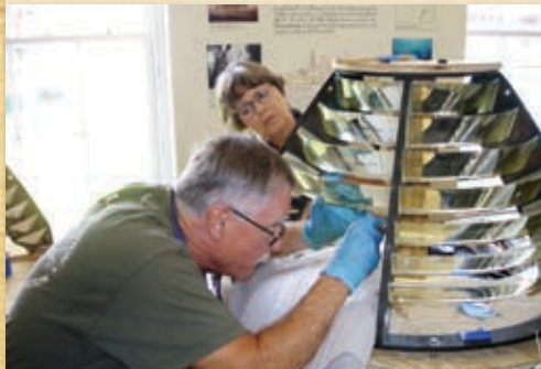
JOHN AND JACKIE MANN REMOVE OLD GLAZING FROM LENS
