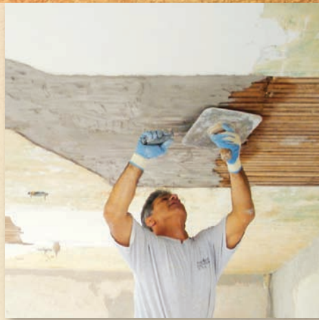
ED MILANO MAKES A CEILING REPAIR
