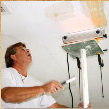
STEVE LINKFIELD USES AN INFRARED PAINT REMOVER ON THE CEILING.
