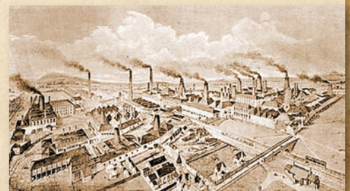
CHANCE BROTHERS GLASSWORKS, NEAR BIRMINGHAM, ENGLAND
