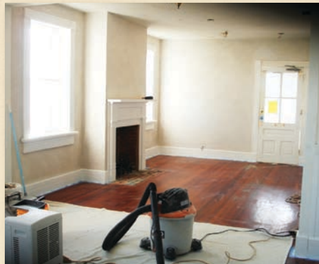
THE LIVING ROOM IS NEARLY COMPLETED.
