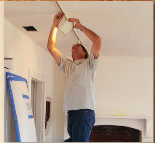
PATRICK SATTERFIELD INSTALLS LIGHTING IN THE COMPLETED ROOM.
