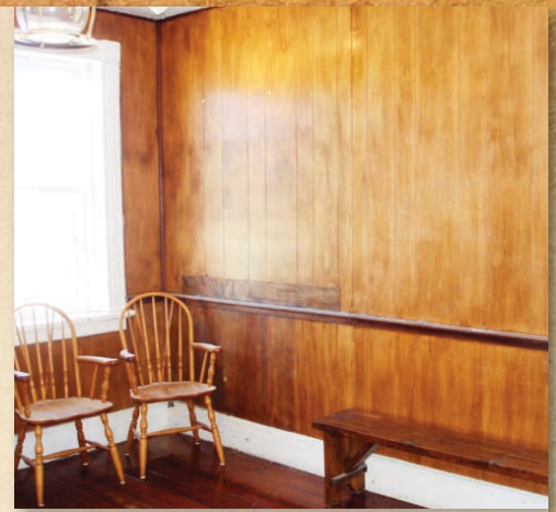
MODERN PANELING HAD TO BE REMOVED.
