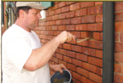
Chuck Spitznagel demonstrates repointing at the Light Station.
